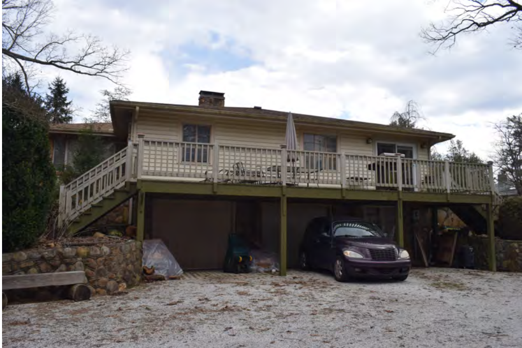
Figure 42: Rear of Cureton House, View to the East-Southeast
