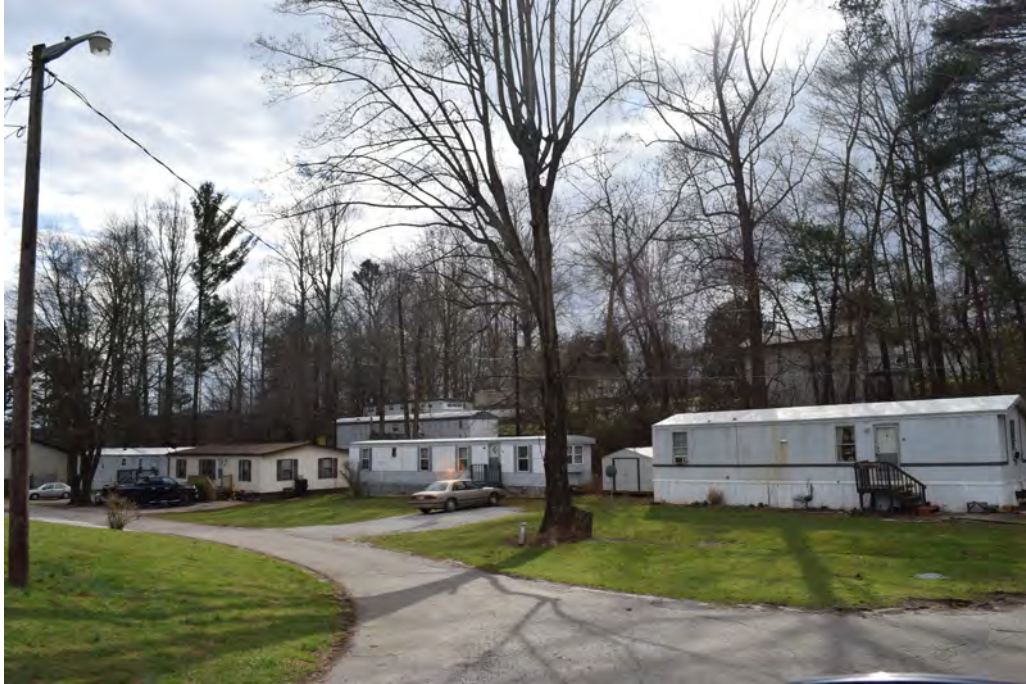
Figure 32: Mobile Homes at 38, 48, 62 and 74 Alverson Lane in Mobile Home Park, View to the Southwest
