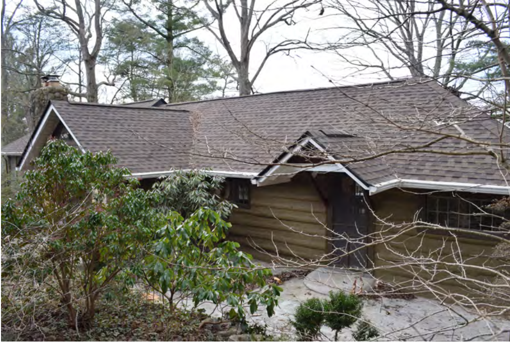
Figure 28: 41 Bicknell Place, 1917 Log Cabin on North End, View to the Southwest
