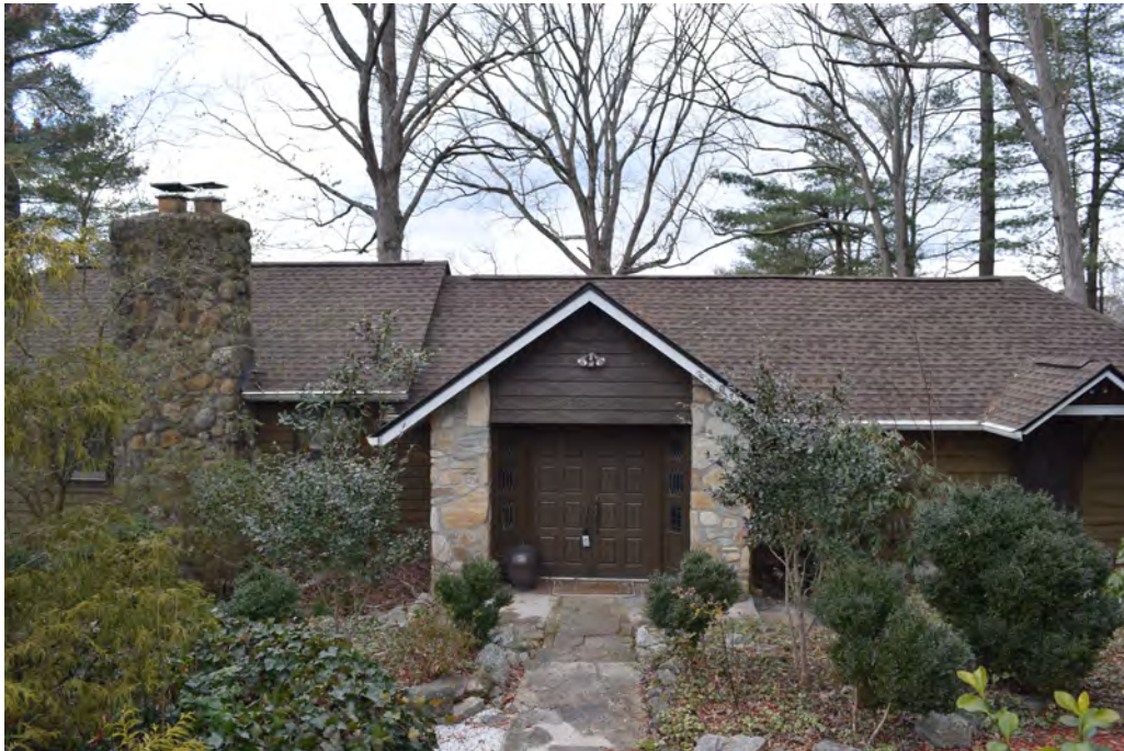
Figure 27: 41 Bicknell Drive, View to the West-Northwest
