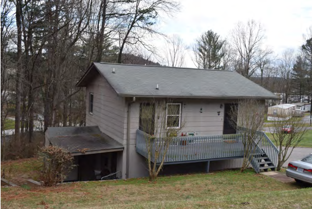
Figure 14: 51-53 Cureton Place, View to the East-Southeast
