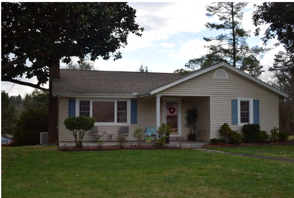
Figure 19: 72 Cureton Place, View to the Southwest
