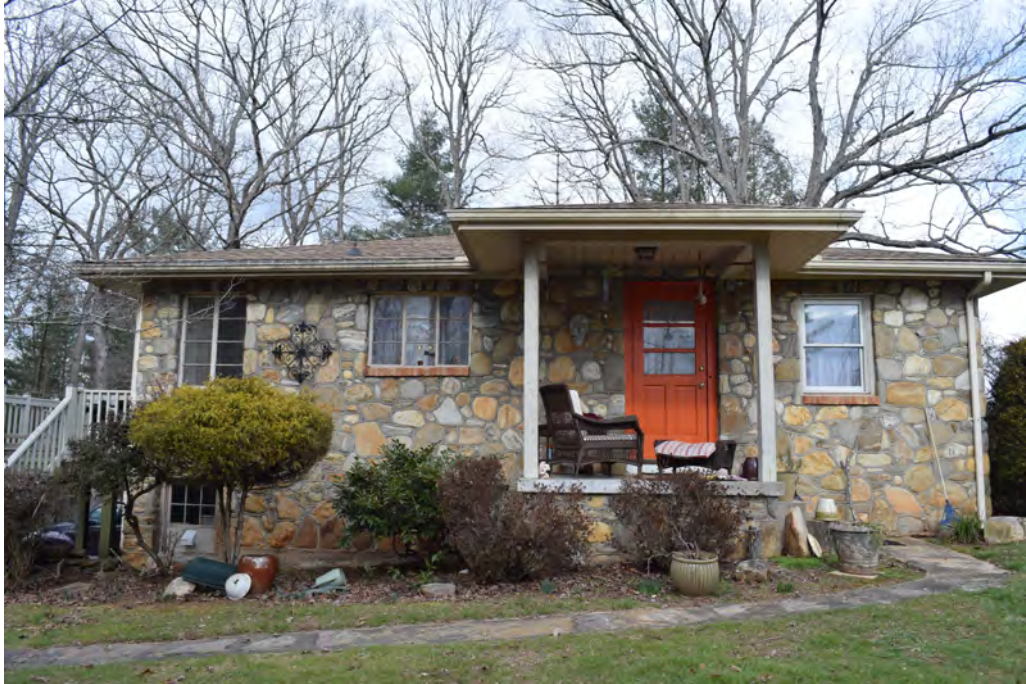
Figure 40: South End of Cureton House, Facing North-Northeast
