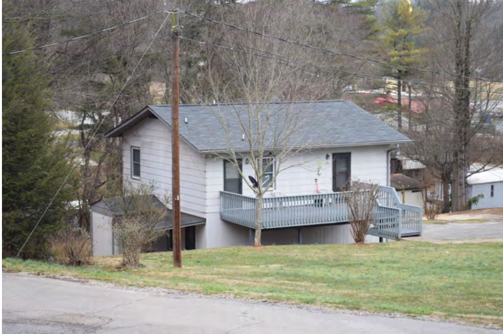
Figure 18: 61-63 Cureton Place, View to the Southeast
