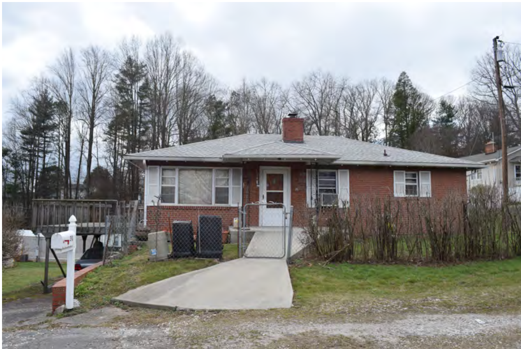
Figure 11: 31 Cureton Place, View to the Southwest
