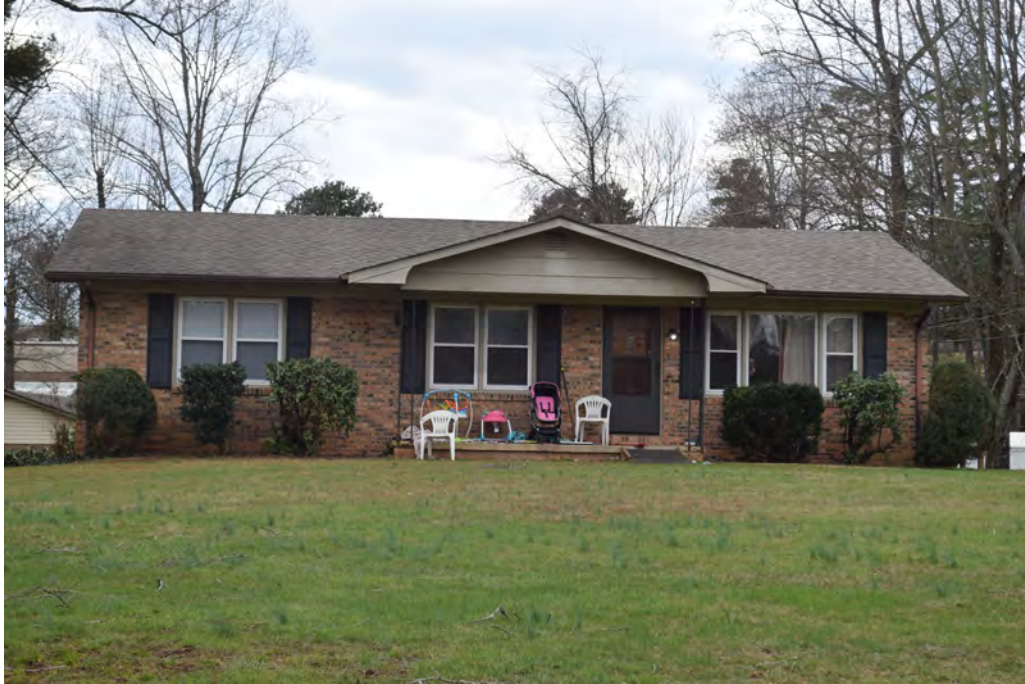
Figure 30: 53 Alverson Lane, View to the Southwest
