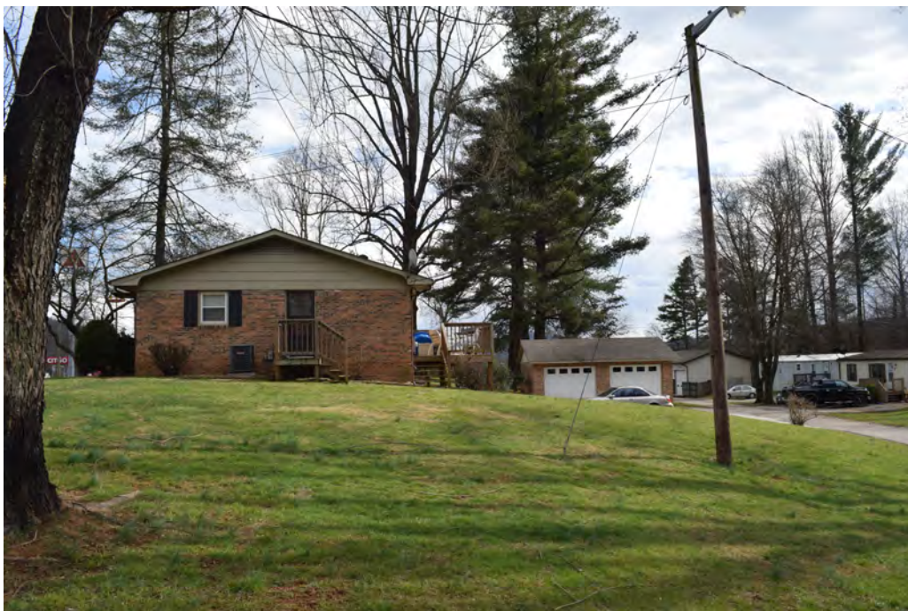
Figure 31: 53 Alverson Lane, Garage to the Right, View to the Southeast
