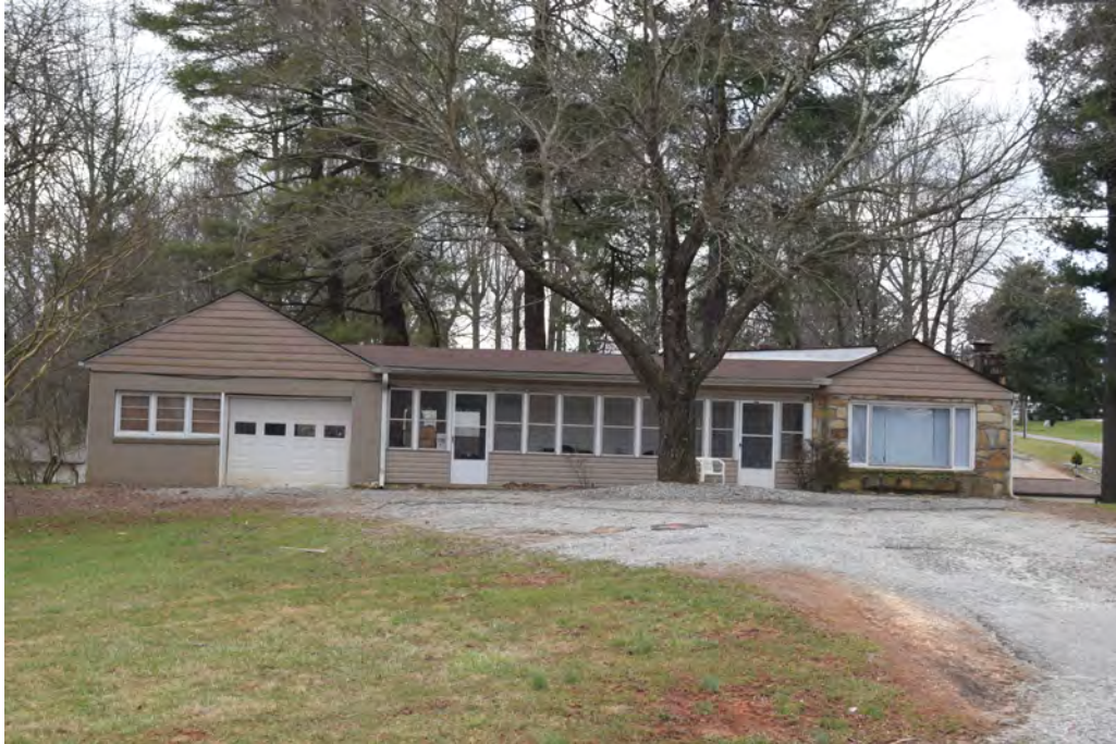
Figure 10: 13 Cureton Place, View to the Southwest
