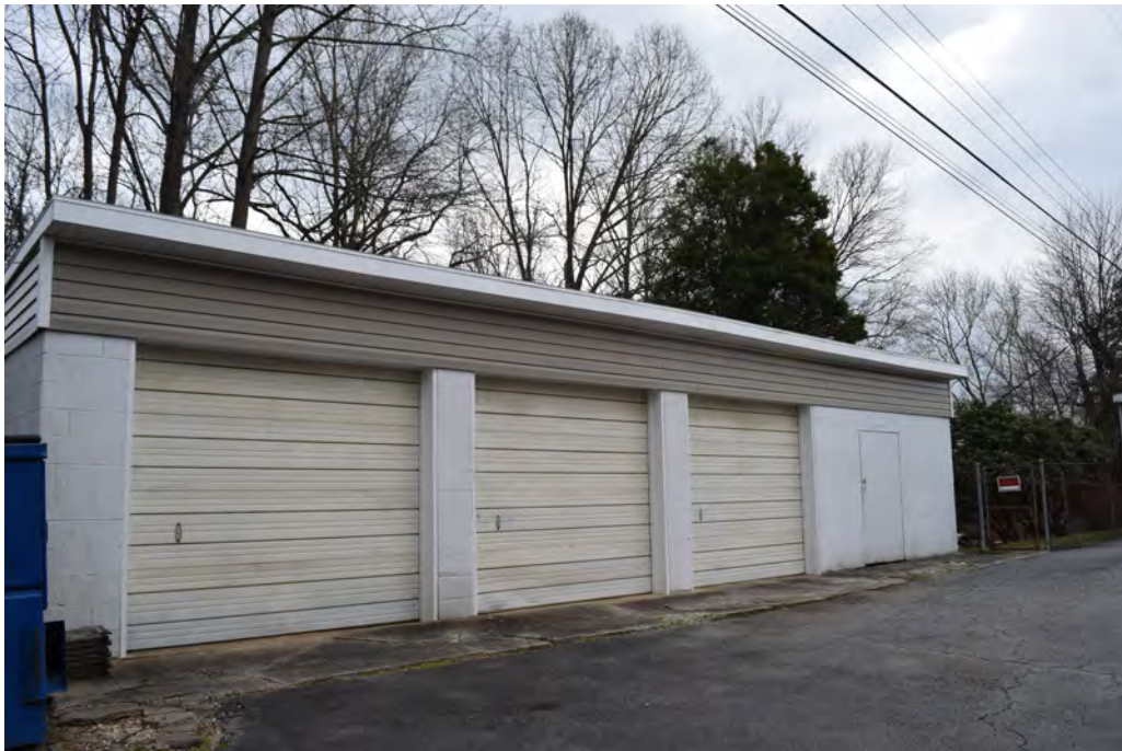
Figure 21: Garage at 76 Cureton Place, View to the South
