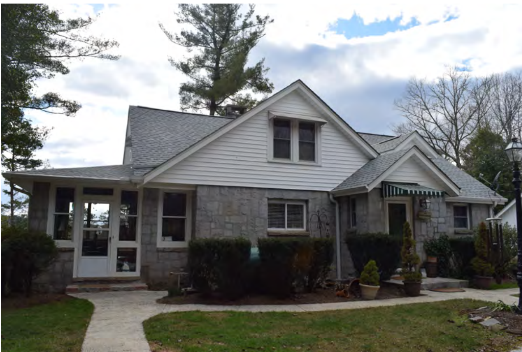
Figure 15: Anne and Carl Stein House, 56 Cureton Place, View to the South
