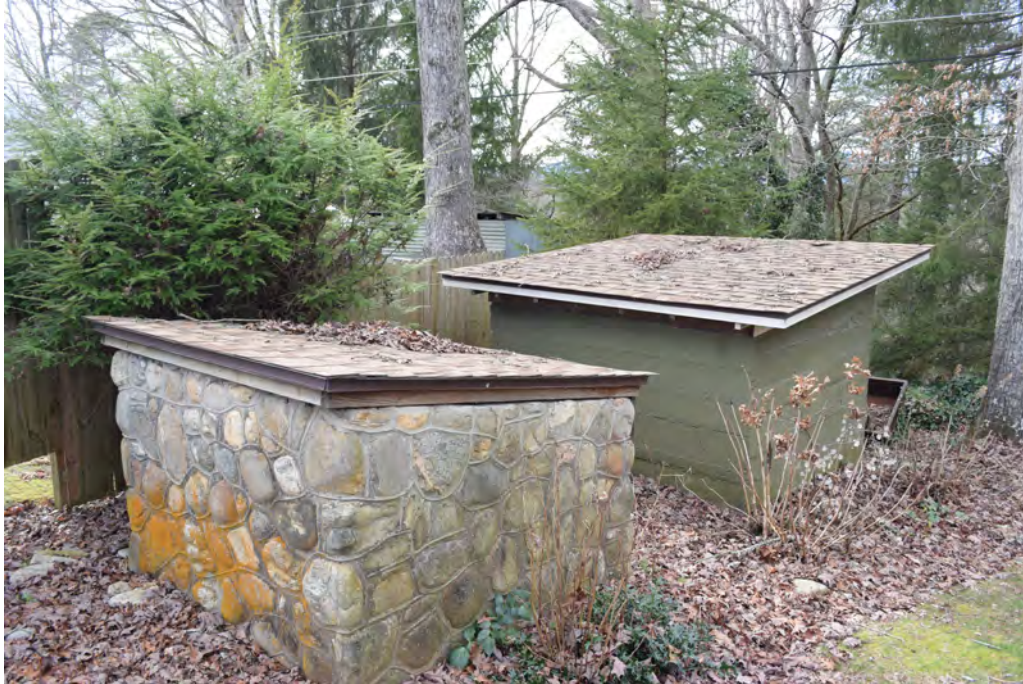
Figure 44: Well Houses in Southwest Yard of Cureton House, View to the Southwest
