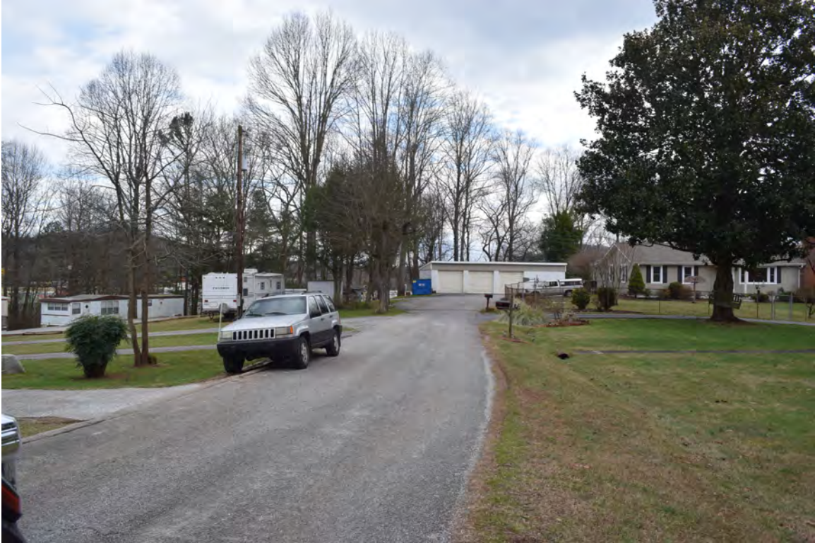
Figure 6: View of Cureton Place, Facing South Toward 76 Cureton Place
