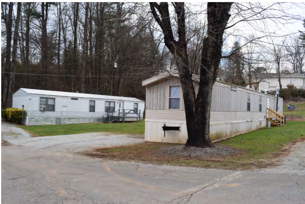
Figure 33: Mobile Homes at 30 and 34 Alverson Lane in Mobile Home Park, View to the West-Northwest
