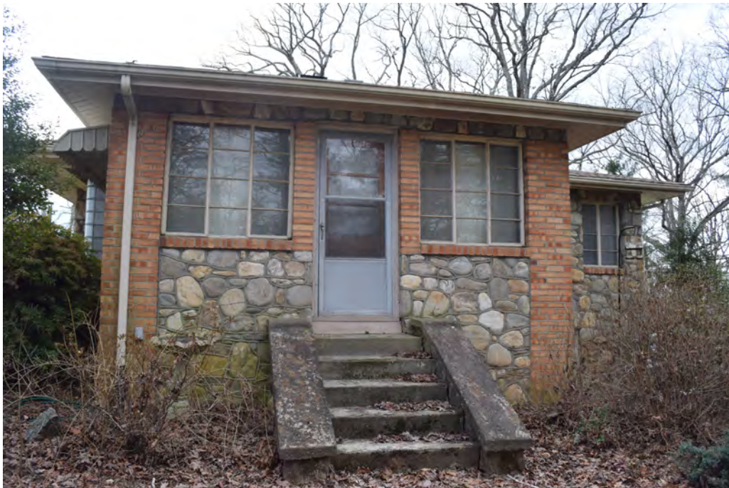
Figure 41: North End of Cureton House, View to the South-Southwest
