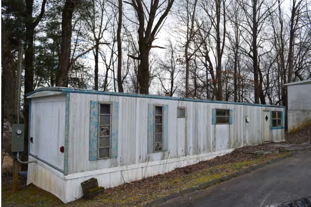
Figure 24: 77 Cureton Place (on same parcel as 76 Cureton Place), View to the South
